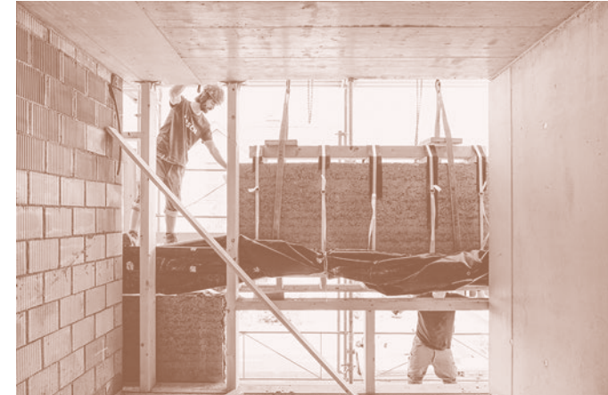
Fig. 22. Construction site scenes with industrialised rammed earth modules on Groffeldstrasse in Buchs.
