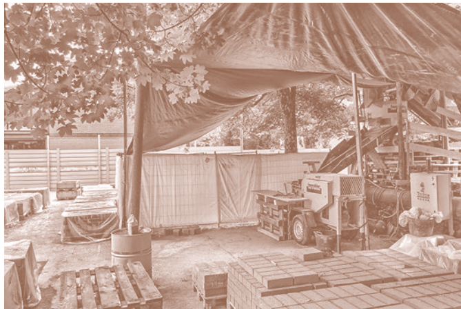
Fig. 23. On-site production of compressed earth blocks.
