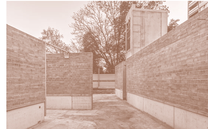
Fig. 24. Load-bearing interior walls at the Geisendorf School, designed by architect David Reffo.
