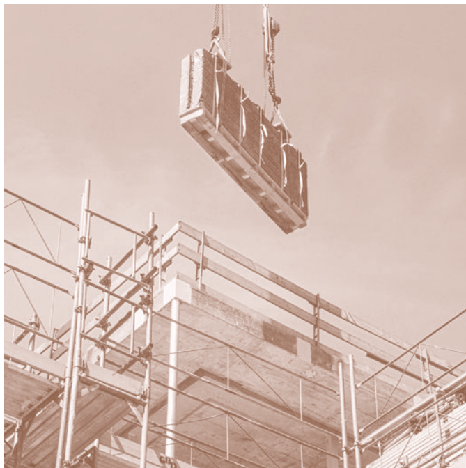
Fig. 21. Construction site scenes with industrialised rammed earth modules on Groffeldstrasse in Buchs.
