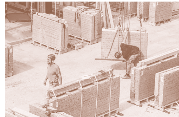
Fig. 20. Construction site scenes with industrialised rammed earth modules on Groffeldstrasse in Buchs.
